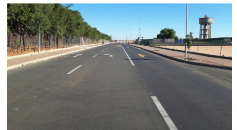
Legogo Road During Construction
