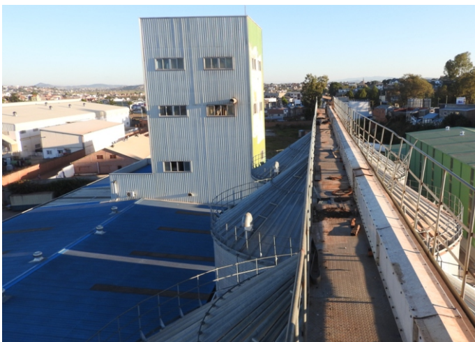
Existing Mill Building and Warehouse
