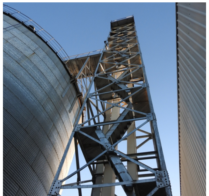
Silos and Elevator Tower
