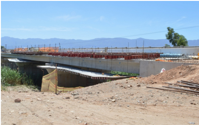
Kogmanskloof Bridge Widening: Working Platforms Suspended from Above Photos courtesy of Eldrid Struis
