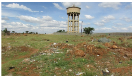
Water Tower Link Road Before Construction
