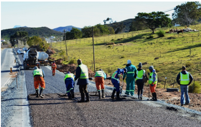
Cape Seal Coarse Slurry Application
