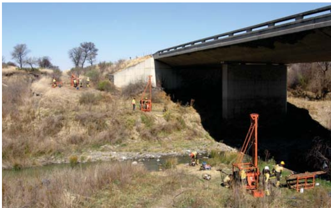
Core drilling for N1 Koppies
