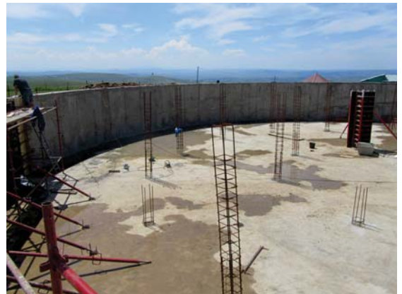
Construction of 2 Ml balancing reservoir
