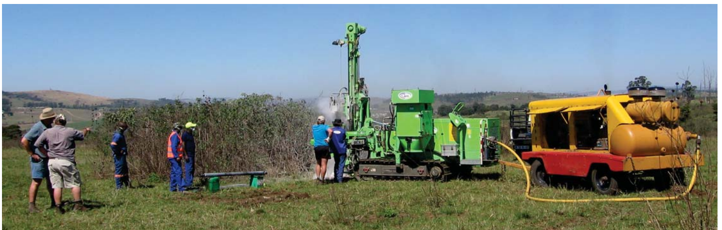
Percussion drilling for N3 quarries
