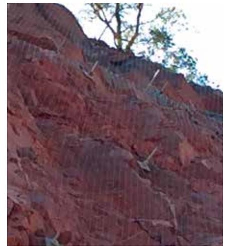
Contractors Guncrete (currently Guncrete Geotechnical), opted to use Geobruigg's Deltax G80/2 mesh. Deltax mesh has lower installation cost as compared to commercially available double twisted mesh. At only 76 kg per 117 m<sup>2</sup> roll of mesh (hexagonal mesh is more or less 164 kg for the same size), the mesh rolls can be handled by hand with only a few workers.
